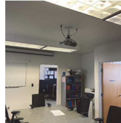
T8 Troffers and older technology systems can be seen in the image above.
