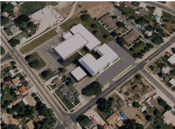
Phase 1 would include construction of a new Community Services Building on the west side of the site.
