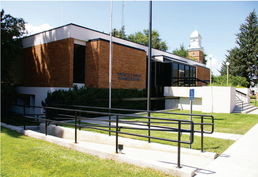
Exterior images illustrate building materials, entry stairs, and ADA access ramp down to lower level at entry.
