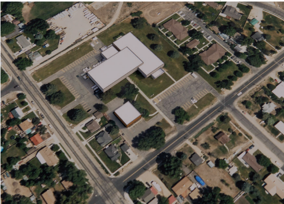
The site currently houses the Community Services and Central Operations buildings.
