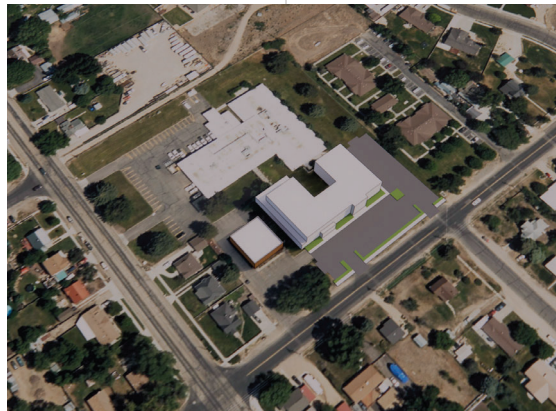
Phase 2 would be the demolition of the old Community Services Building.
