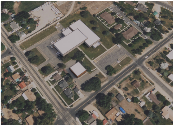
The site currently houses the Community Services and Central Operations buildings.
