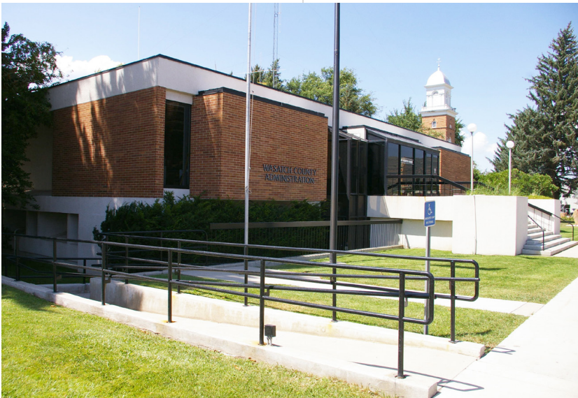
Exterior images illustrate building materials, entry stairs, and ADA access ramp down to lower level at entry.
