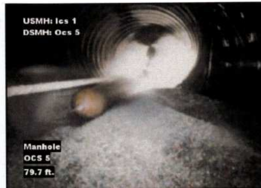
Cleaning Separator Row and pipes with high pressure water nozzle
